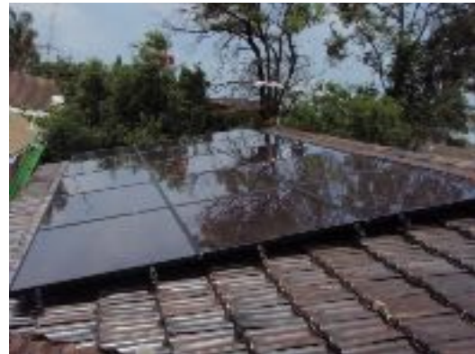
Solar hot water panels of dry design
