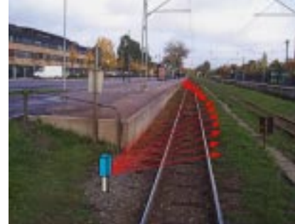
Alarm system for people walking on the rail tracks in a station
