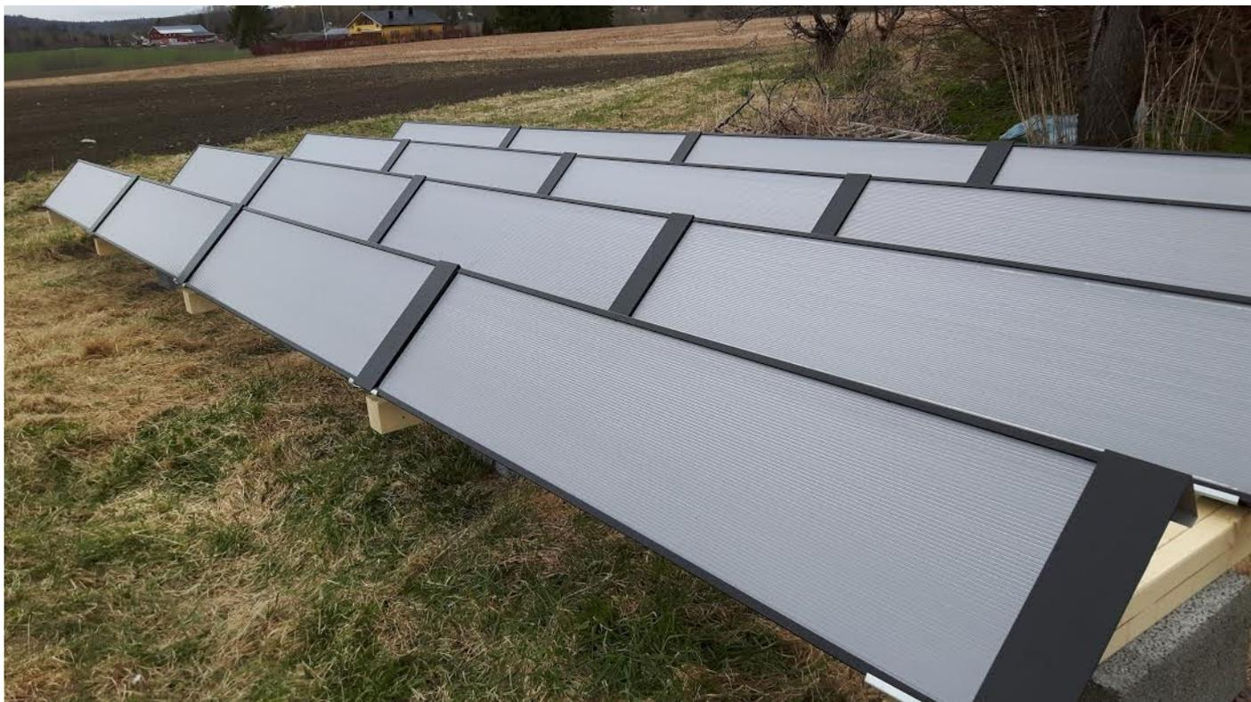
SF 800 is a solar hot water thermal panel designs to use solar radiation to get hot water. It is vert straight and sold design produced in Norway. Unique is it is a design where no antifreeze is needed when cold. It have self drain solution that makes installation far better and no unhealthy antifreeze is needed. It is made in aluminium with Poly carbonate window that is a special opaque design to preserve heat inside
