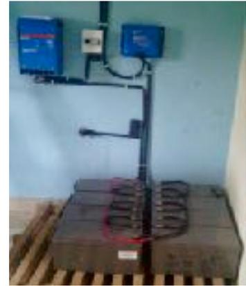
2017 we installed a solar system for illumination at Maison Dorcas in Bukavu Congo. This is related to the Panzi hospital group. Here we make a stand alone system for 250 Pcs led lamps we delivered to get power at nights when god is down . Panels are of the new cloudy weather design as Bukavu is not very sunny.
