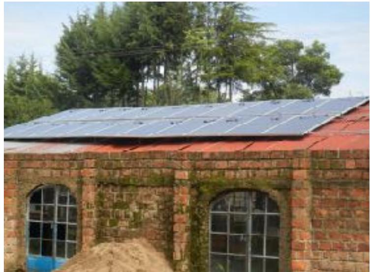
**Dormitory system in school Kenya** 2014 we installed about 20KW solar panels and a battery system of almost 100KWH in Kericho in Kenya. System handle a dormitory of 700 students with 100% of energy needs. We use 250 W solar panels combined with the 931 AH OPZV battery by North Star. Photo show 1 set up of panels of 12.5 KW and battery back up system. Inverters are 3 Phase 2X12 KW output with MPPT chargers. This system is now working (2017) with zero maintenance and customer is very happy.
