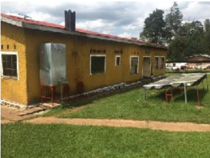
Kiremba Orphanage. 2015 we installed hot water systems in 8 houses at an orphanage for baby This includes a larger system at then kitchen and smaller systems in each small house. Here we save lots of wood as well as electricity. Old grid was very unreliable and often knocked out. Now all works far better. The tank at kitchen is 500 Liter and made in Sweden as well as panels. Each panel gives about 1.5 KW thermal power. Now we have installed 18 units of thermal
